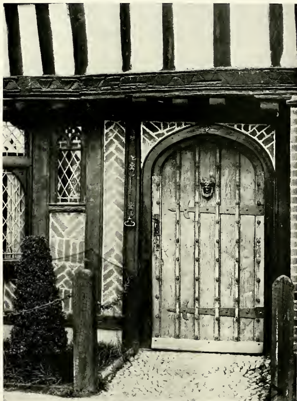
ENTRANCE DOOR, HOUSE AT ARDLEIGH
